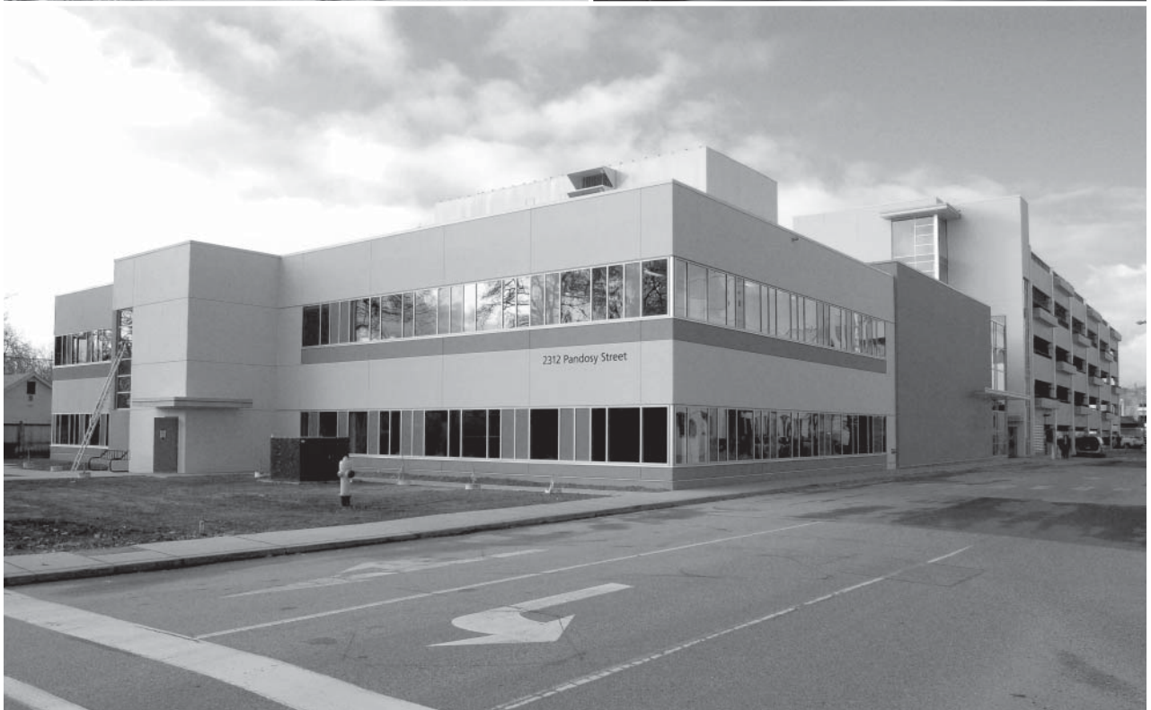
Clockwise from top left: Vernon Jubilee Hospital Patient Care Tower; site excavation for the Kelowna General Hospital Patient Care Tower; Kelowna General Hospital Patient Care Tower; University of British Columbia Clinical Academic Campus
