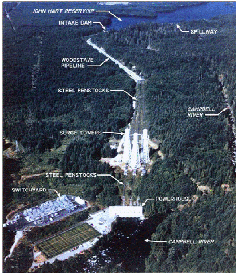
Figure 1: John Hart Facility
